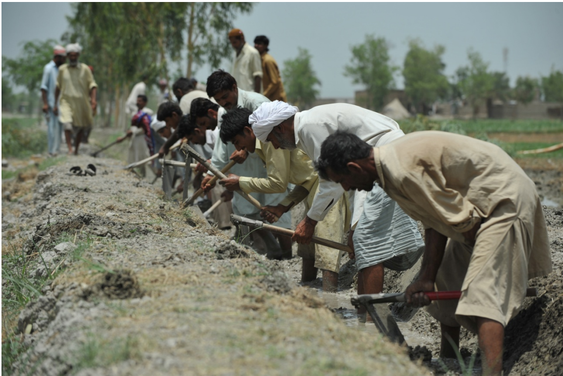
Photo: FAO cash-for-work beneficiaries repairing irrigation infrastructure after the 2010 floods in Pakistan
